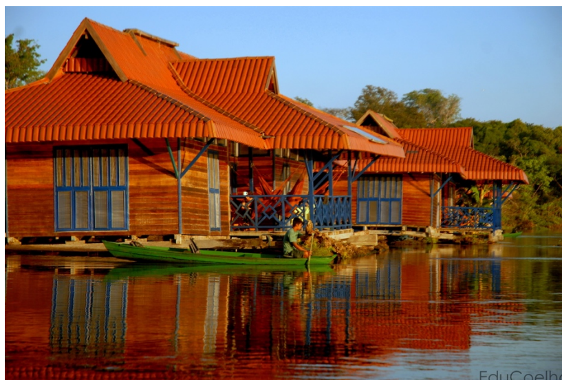
Image 02: The floating structure of Uakari Lodge from the water level. (Credits: Eduardo Coelho)
